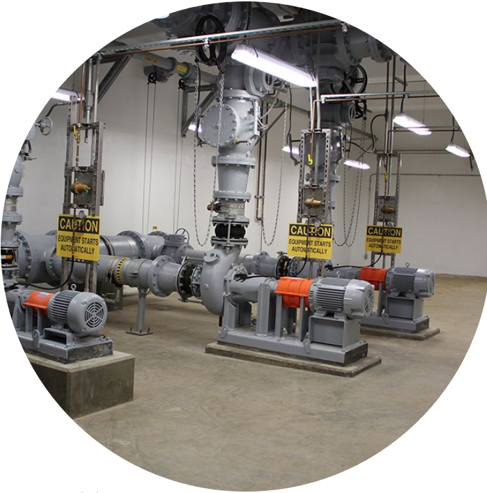
New Return Sludge Pump Station serving the new third treatment train with space for a future fourth train.
