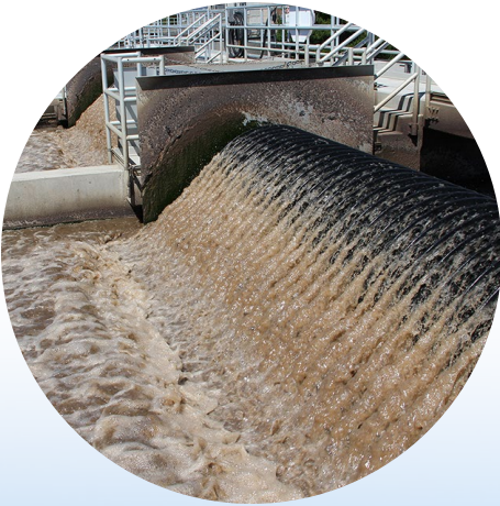
Optimized aeration basin matching the size of the existing basins but with an additional 10-percent treatment capacity.
