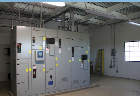
Translucent wall panels
