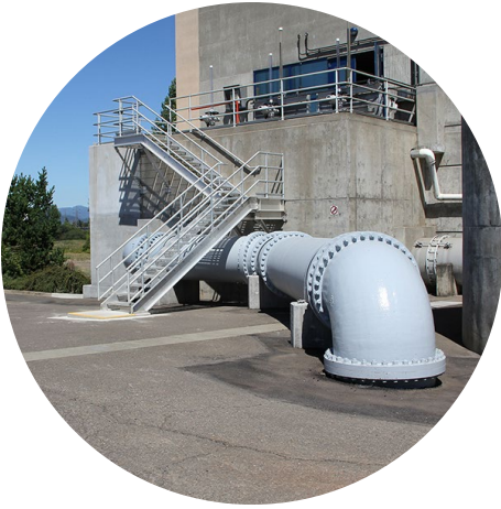
42-inch diameter ductile iron pipe added to the existing Headworks to split flow to the new aeration basin.
