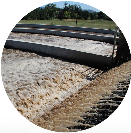
Oxidation ditch aeration basin with three zones.
