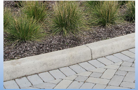
Extensive permeable paver and landscaping design by Greenworks minimizes stormwater runoff to the Yamhill River.
